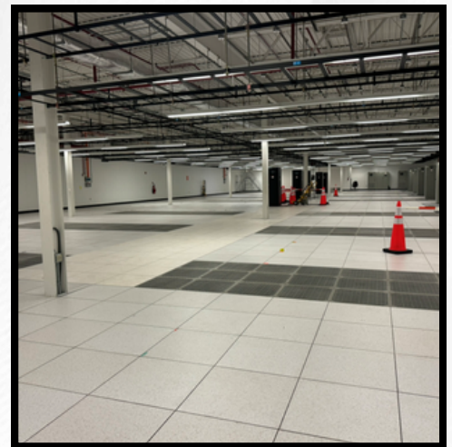
Space redesigned for electrical and mechanical infrastructure requirements
